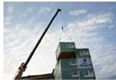
Figure 1: Prefabricated volumes are easily and quickly mounted at the building site
